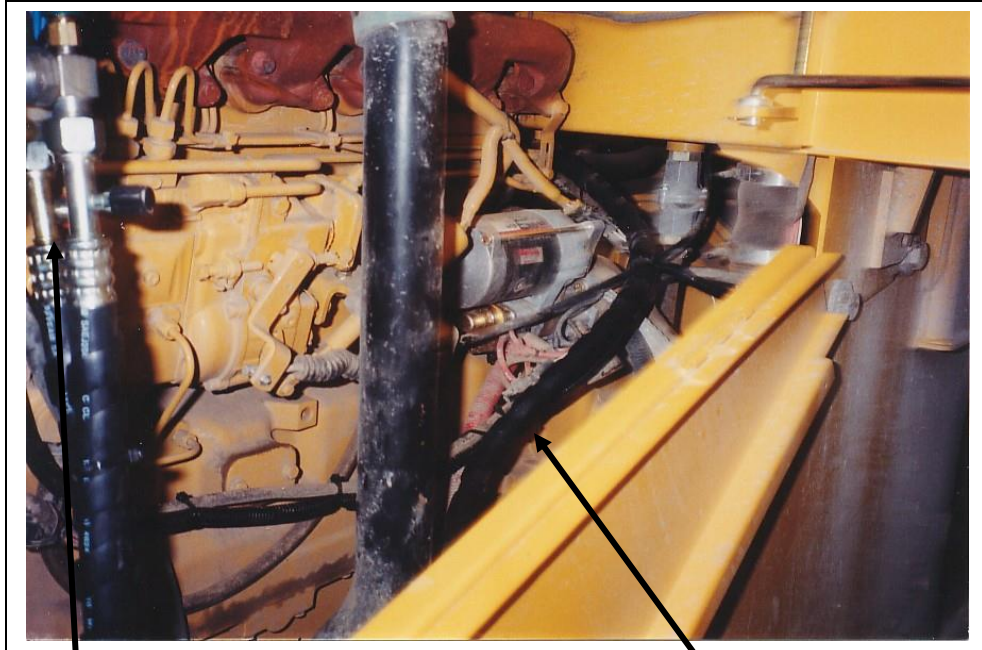
13/32" hose running towards the top fitting on the condenser
